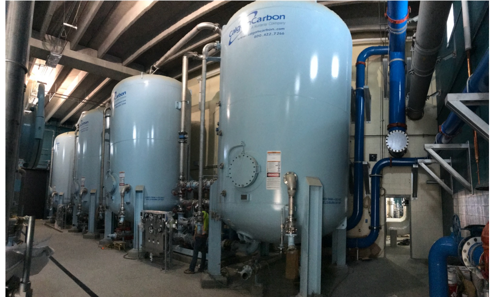
Granular Activated Carbon Filters at Plum Creek Water Purification Facility
