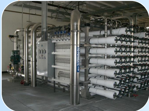
Chino II Desalter Expansion
