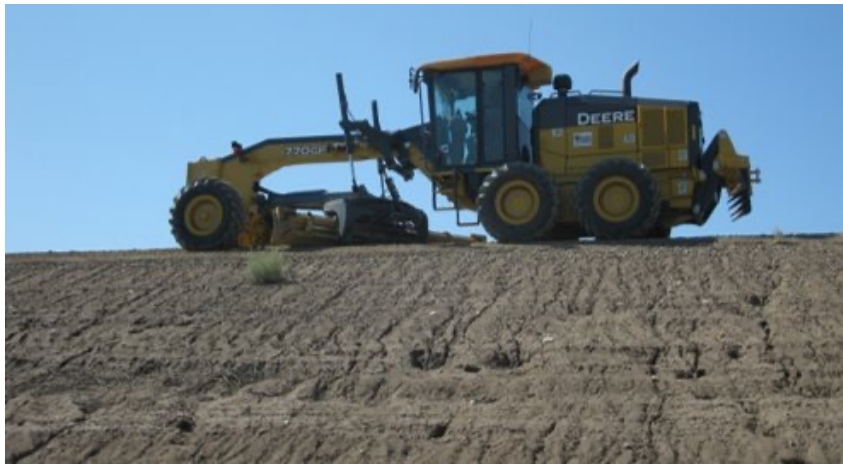
Equipment on the levee
