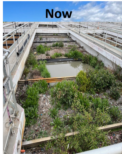
Primary Sedimentation Tank in San Diego
