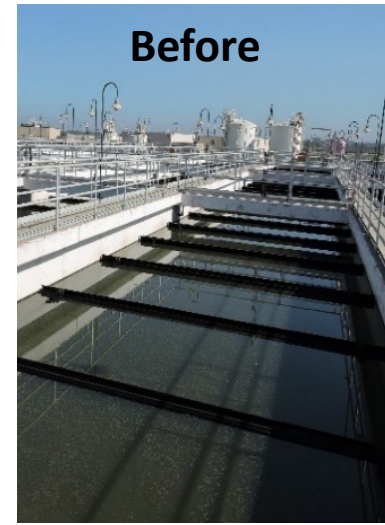
Primary Sedimentation Tank in San Diego
