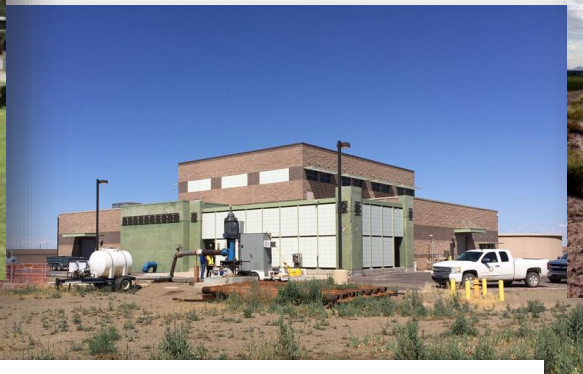
Surface Water Treatment Plant
