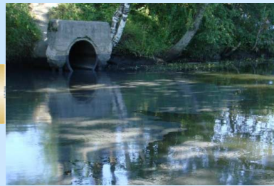
Discharge to River
