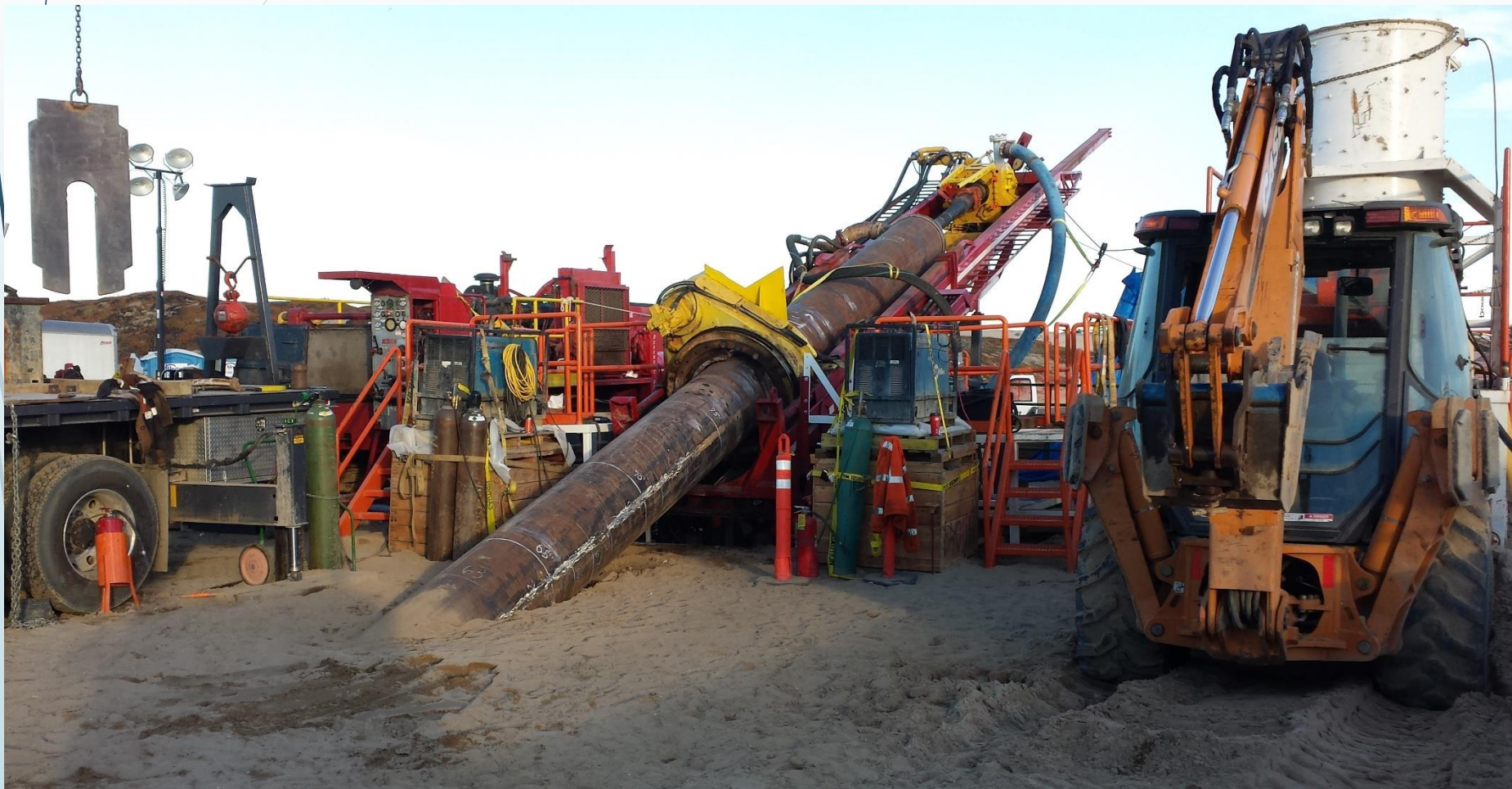
DR-40 Slant Drill Rig
