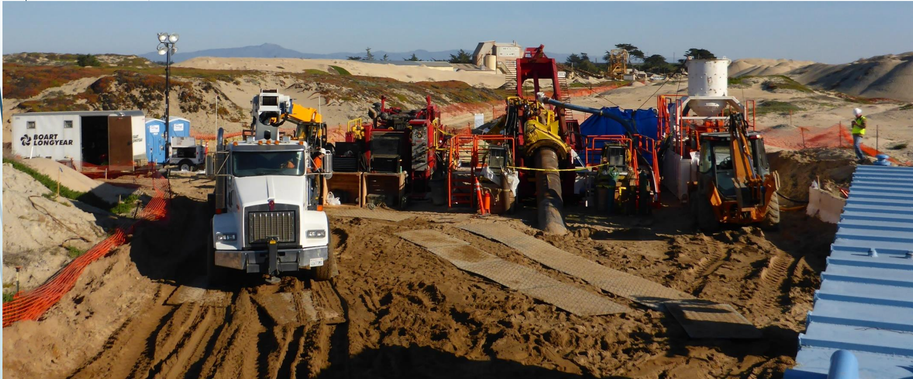
Typical Equipment Required at Drilling Site
