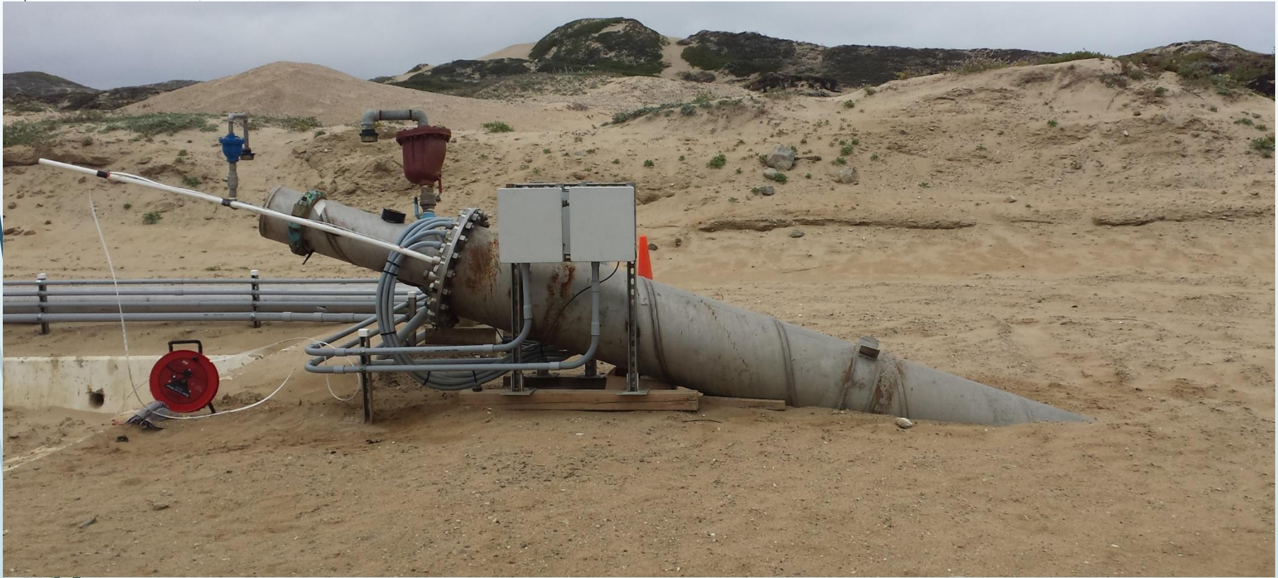
Completed Test Slant Well
