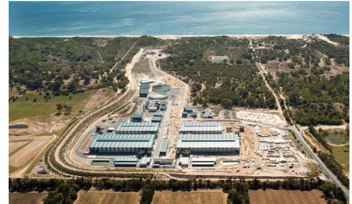
Perth Binningup Plant 60MGD 2013
